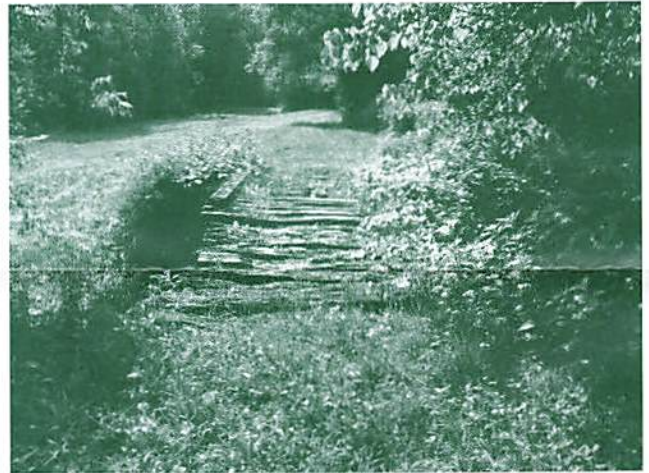
The bridge prior to reconstruction
