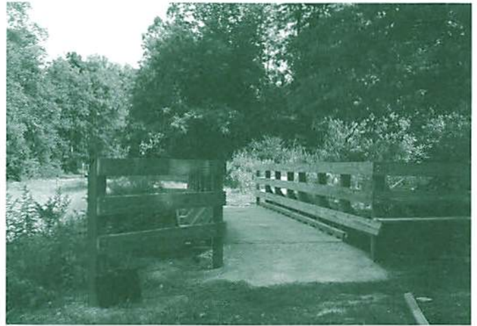
Completed bridge, which involved over 375 man- hours of work.
