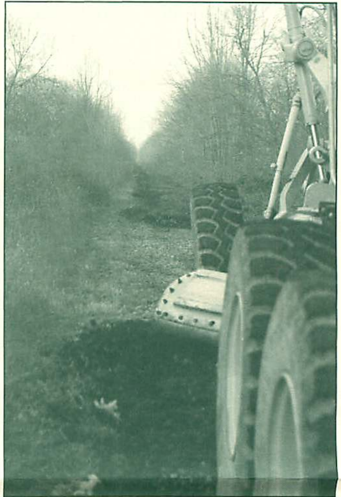
Road grader beginning to grade trail surface
