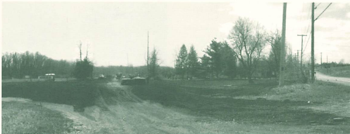
Phase 1 of the Parking Lot Improvement Project is underway.
