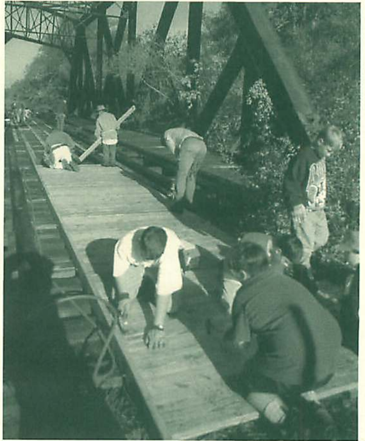
Trestle bridge over Honeoye Creek
